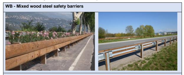
**Description**: Combined wood and steel guardrails adapted to natural sites, ensuring aesthetic continuity. These types of barriers are in accordance with EN-1317 European standards.
