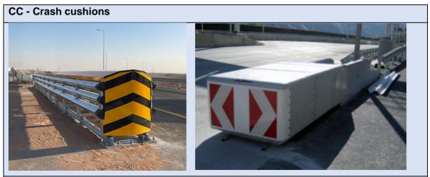
**Description**: Crash cushions are a road vehicle energy absorption device installed in front of rigid objects to contain and redirect a vehicle (i.e. redirective crash cushion) or to contain and capture it (i.e. non-redirective crash cushion). Crash cushions are tested in accordance with EN 1317-3.
