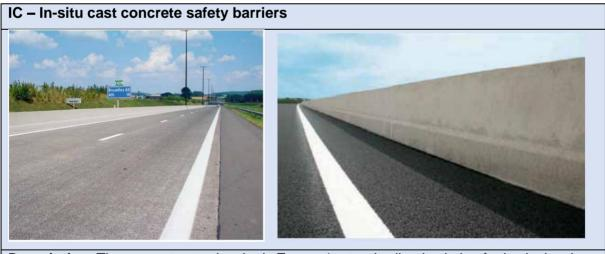
**Description**: The concrete step barrier is Europe 's standardised solution for in situ barriers. The concrete barrier is poured on site, situated directly on the road, with the use of slipform machine by means of a mould.
