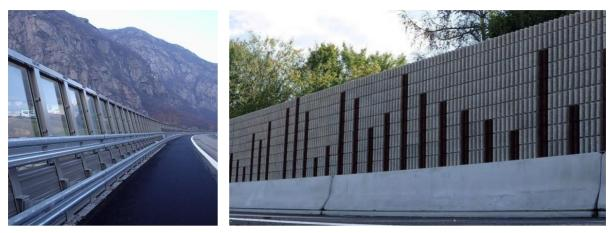
Figure 2: Different types of integrated noise and safety barriers of different materials in Europe (steel & transparent left side and fully concrete type right side).
