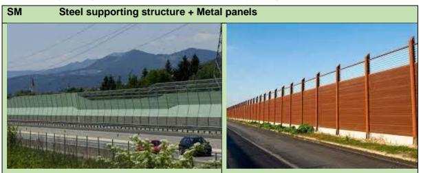
**Description**: noise barrier made of structural elements (steel posts + base plate and anchor bolts) + acoustic elements made of a metallic cassette (steel or aluminium) with an inner sound absorbing material (rockwool, glass wool or polyester foam).
