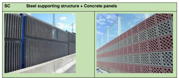
**Description**: noise barrier made of structural elements (steel posts + base plate and anchor bolts) + acoustic elements made of a double layer concrete panel (supporting layer made of steel reinforced concrete + sound absorbing layer made of light concrete, expanded clay, mixed concrete and wooden chips).
