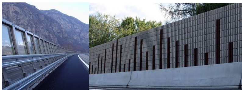
Figure 1: Different types of integrated noise and safety barriers of different materials in Europe (steel & transparent left side and fully concrete type right side).
